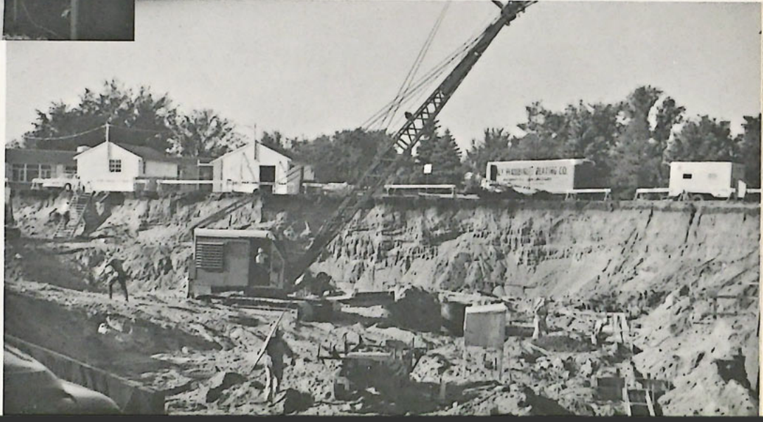
Some indication of the size of the new hospital addition is apparent in the extensive excavation which was required. The new structure will consist of six floors plus a new elevator system to supplement that in the original building.
