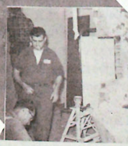
This is the ground work reconstruction
