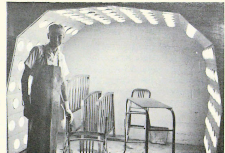
7. The final step in the refinishing process is a drying period in the "auto-bake." Here, 120 infra-red lamps penetrate through the paint to heat the metal, drying the paint from the inside out.
