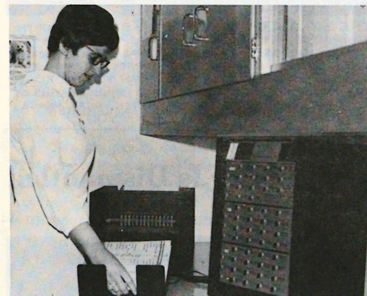
ANNA MAE SUPAN, DIETARY DEPARTMENT MESSENGER, OPERATES THE MENU-MATIC COUNTING DEVICE WHICH ADDS THE VARIOUS ITEMS ORDERED BY PATIENTS FOR THREE MEALS IN ADVANCE, AT THE RATE OF 100 PER MINUTE. THE MACHINE WILL COUNT FIVE TYPES OF DIETS IN 10 MINUTES, PROVIDING CHEFS WITH ACCURATE QUANTITY REQUIREMENTS.
