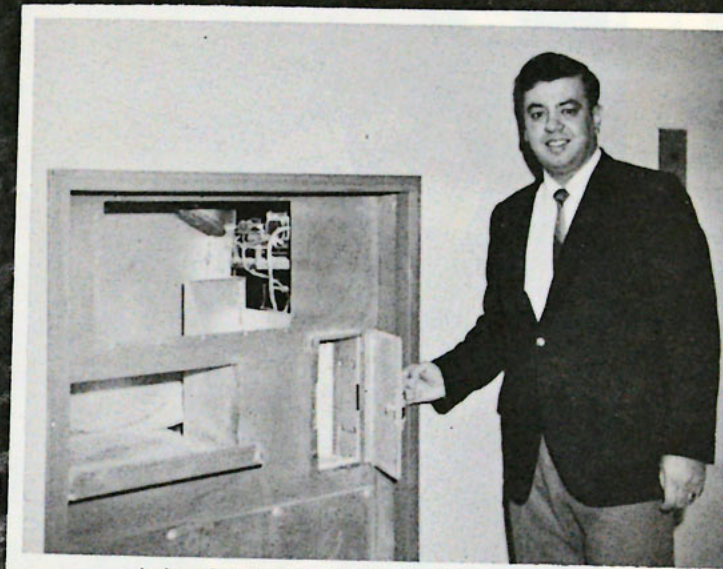
LAMSON TUBE SYSTEM RECEIVING STATION. THROUGH THIS DOOR A TUBE WILL COME OUT WHICH CARRIES A MESSAGE.
