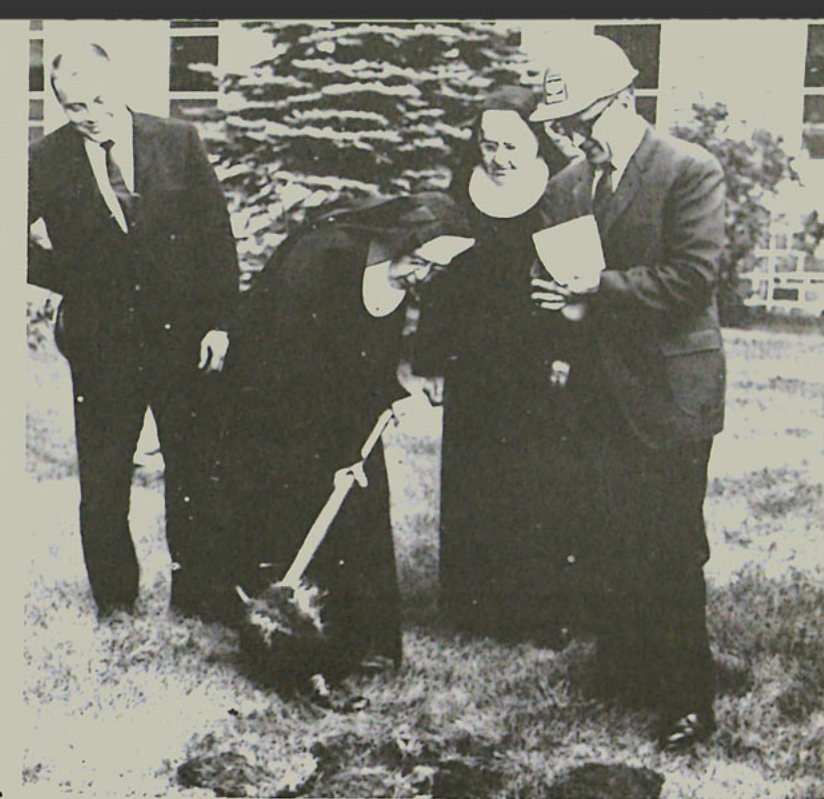
ST. CLOUD HOSPITAL'S FIRST ADMINISTRATOR, SISTER JULITTA TURNED OVER ONE OF THE FIRST SHOVELS OF DIRT IN PREPARATION FOR THE BEGINNING OF WORK ON THE NEW WING MONDAY, AUGUST 5. AT THE LEFT IS DR. JEROME BALLANTINE, CHIEF OF STAFF. AT THE RIGHT ARE SISTER CONSILIA WHO HAS WORKED AT ST. CLOUD HOSPITAL SINCE IT OPENED IN 1928, AND ADMINISTRATOR GENE S. BAKKE.
