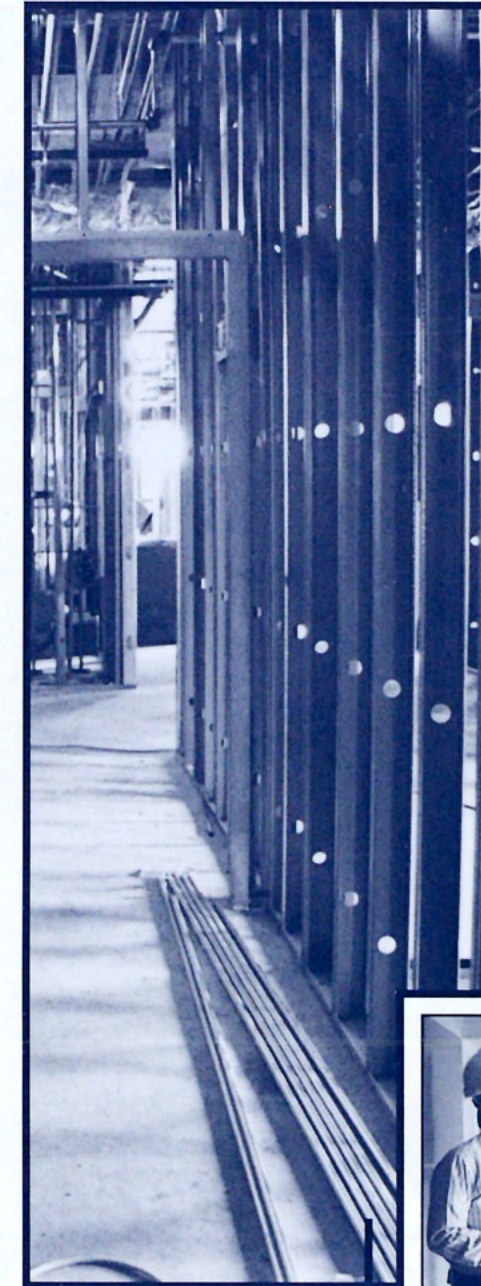
Steel studs line the corridors of what will be the Central Minnesota Heart Center in the South Building being added to the St. Cloud Hospital.
